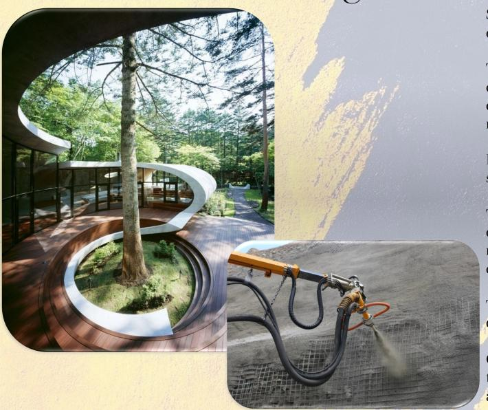
Shotcreting makes building walls and other structures using only one-sided or non-removable formwork possible.
